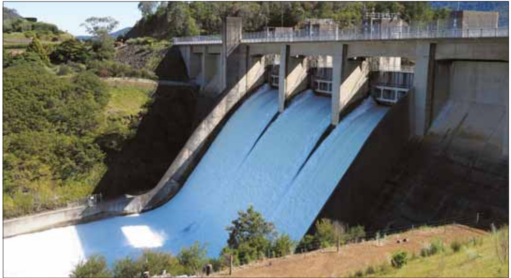
The Lake Eildon spillway. -AR
