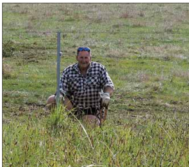
There were plenty of fences needing repairs. -AR
