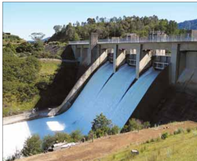
The Lake Eildon spillway. -AR
