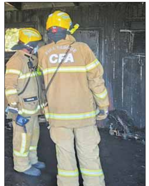
The burnt interior of the house. -S
