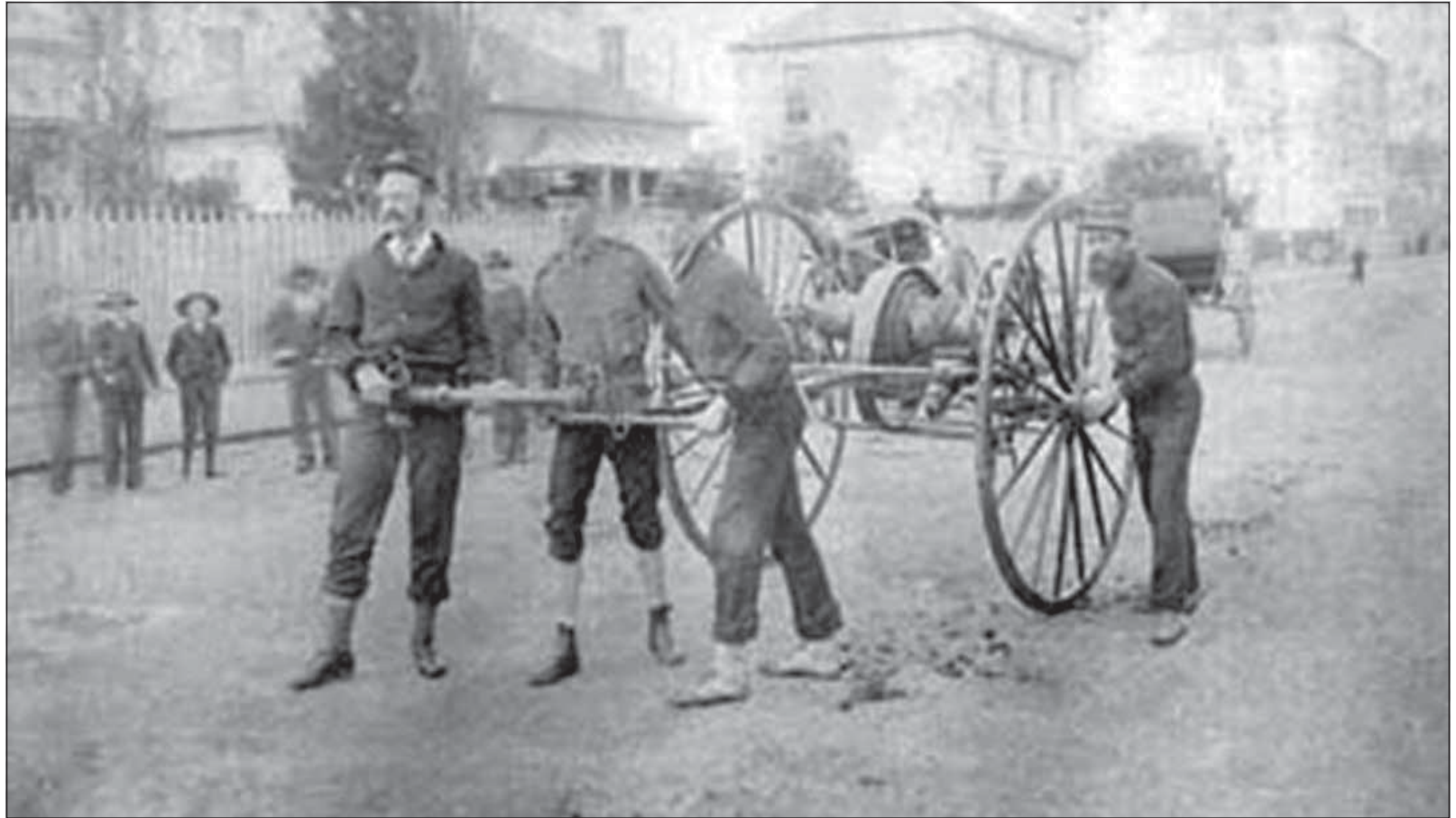
A fire hose on reel which was taken to fires on foot. -S
