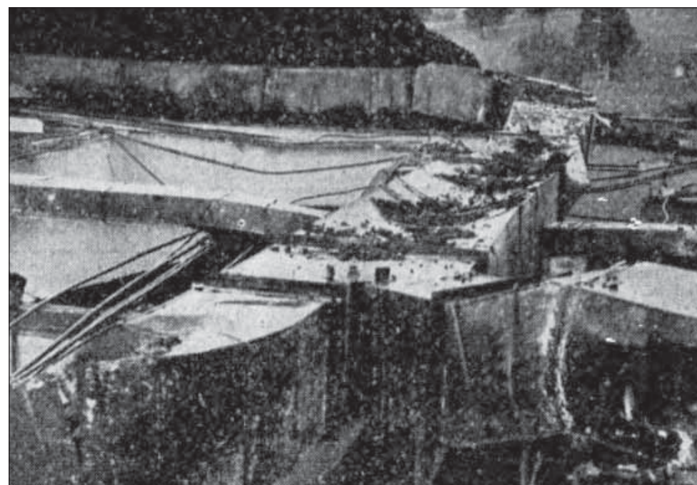
Alexandra's hospital after the fire. -S
