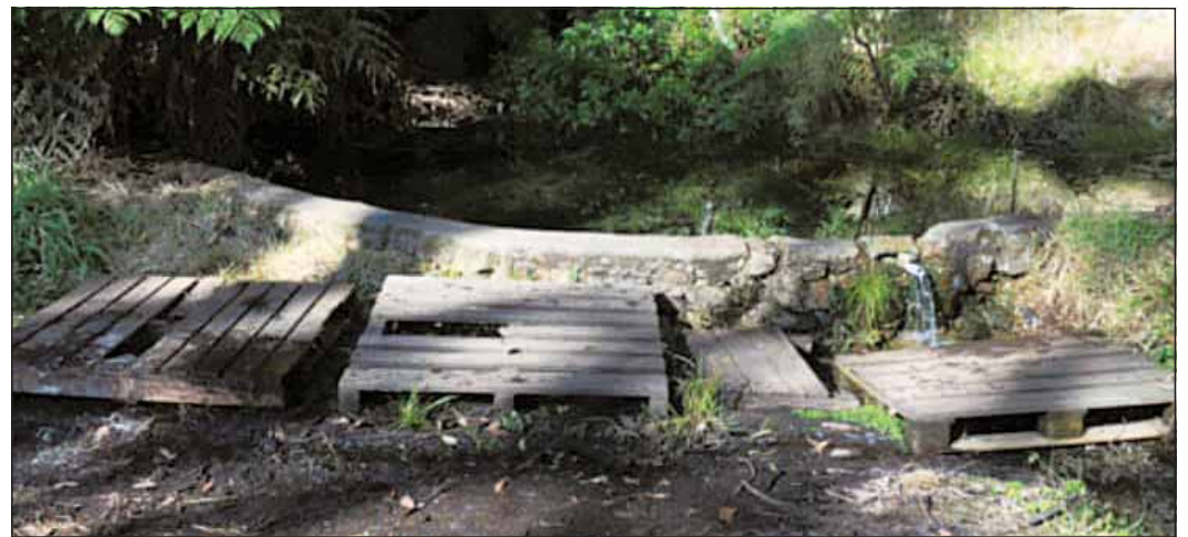
St Ronan's Well prior to the works. -S
