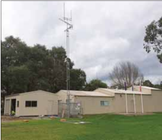
The radio tower that will be removed that was erected after the 2009 Bushfires. - Buxton Fire Brigade
